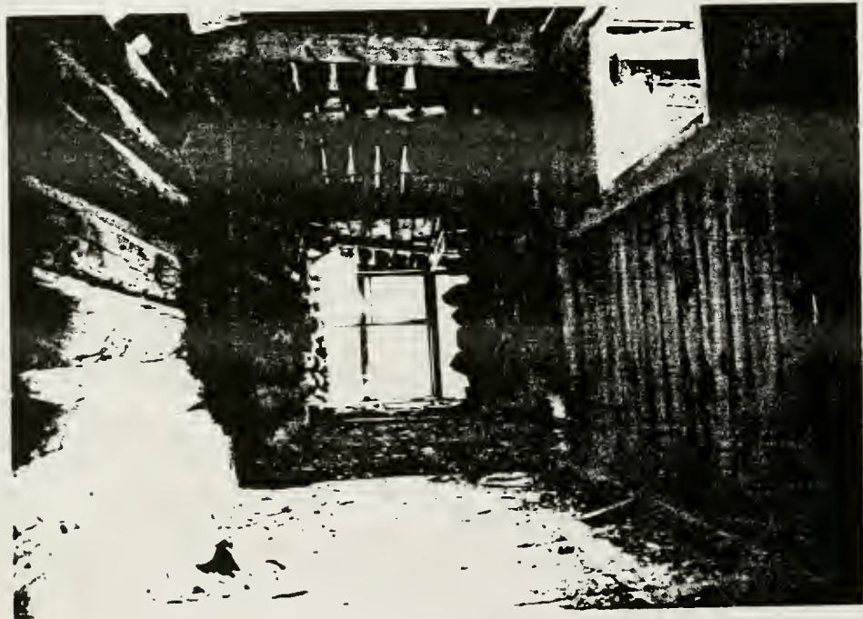
Figure 266. Stuart-Schultz Cabin (24PA410), west view into passageway that is reminiscent of the dog run of early cabins in the southern United States.
